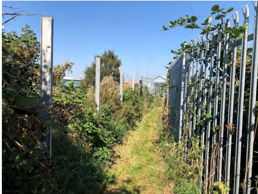
Figure 1-7 Broken sections of fencing and general sense of neglect along the path.
