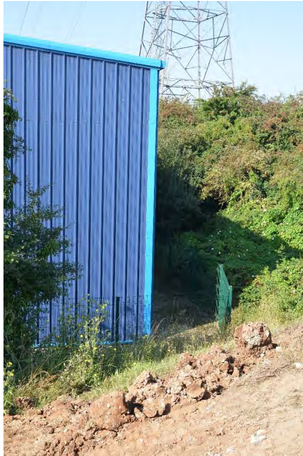
Figure 1-5 Footpath Bost/14/12 does not appear to exist on the ground (view looking west from the northern end of footpath BOST/14/11)
